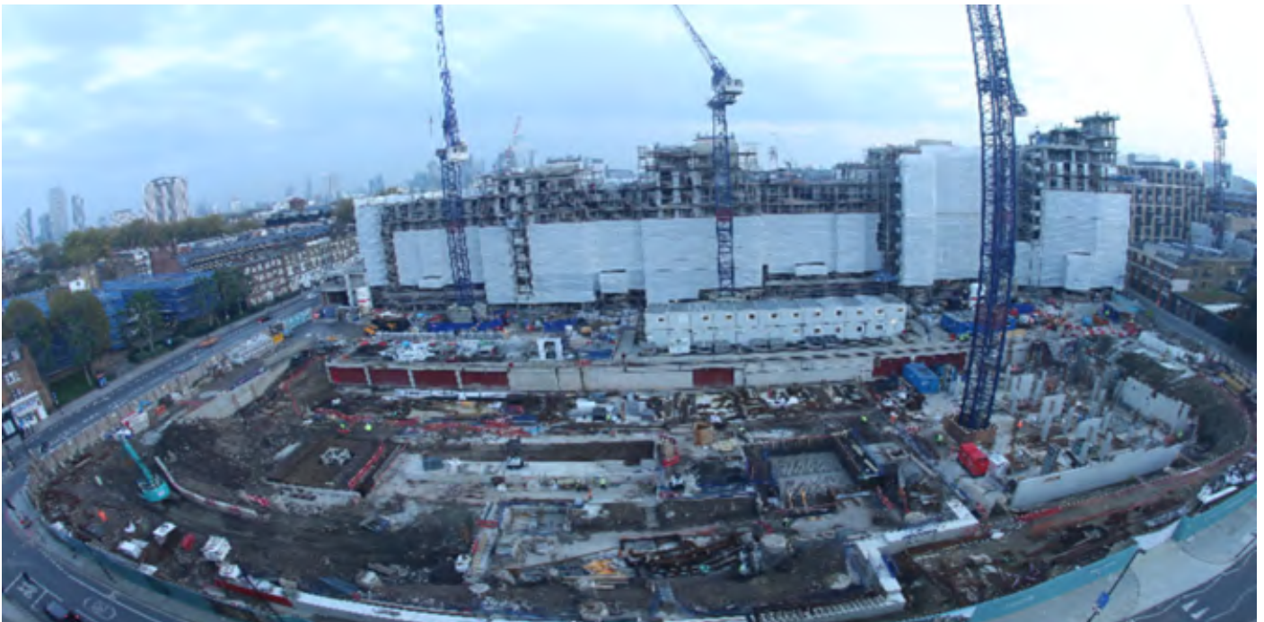
Progress at Phase 3
