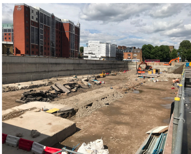
Enabling works for phases 3 and 4
